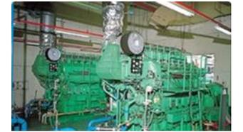
Diesel engines for emergency pumps
